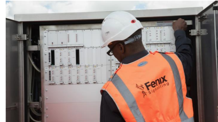
Figure 5 - External location cabinet (frame closed)
