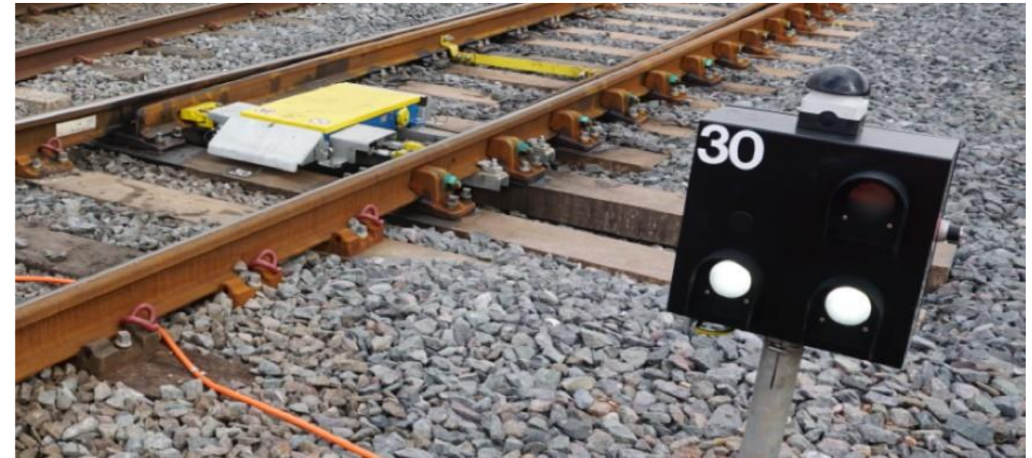
Figure 5 - Points Position Indicator
