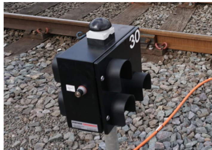
Figure 1 - Plunger mounted on top of PPI (optional) and keyswitch (labelled WHT)
