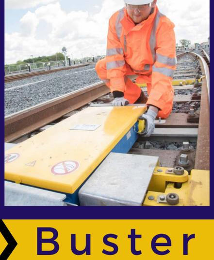
Although not usually a practice in the UK, the machines are trailable, meaning that a move through a set of trailing points set in the wrong position does not damage the machine. There is also only one cable required, unlike most UK mechanisms which require two, as the PT 110i provides the 400V three-phase supply and also the detection in one cable.
