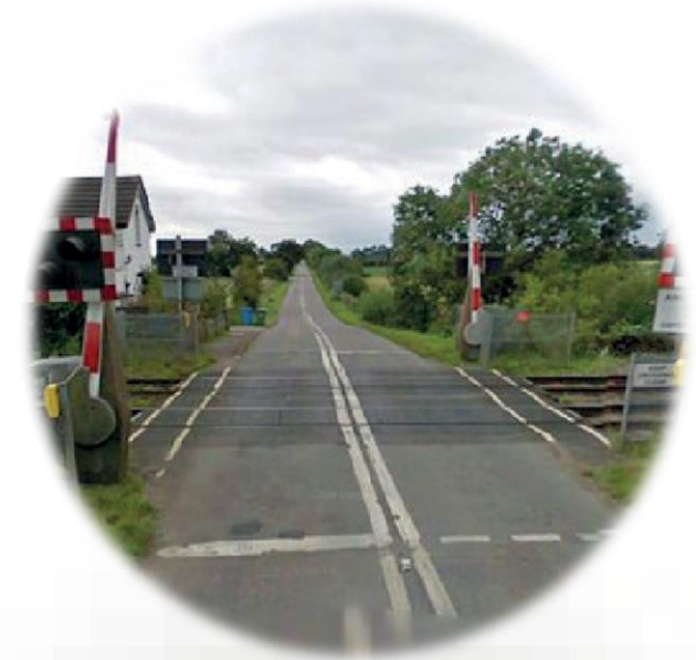
Level Crossing Survey
