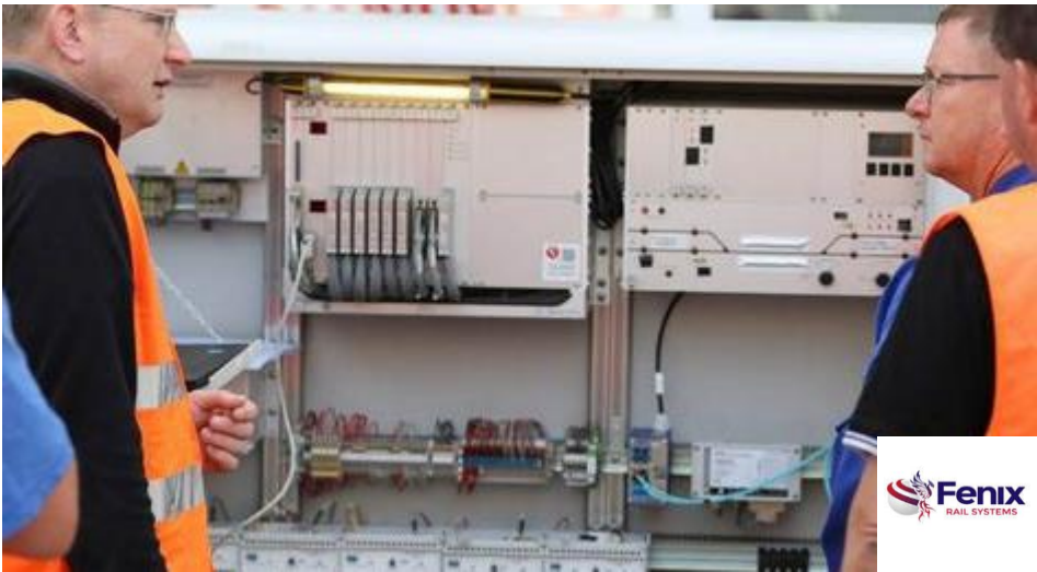
External location cabinet (frame open)
