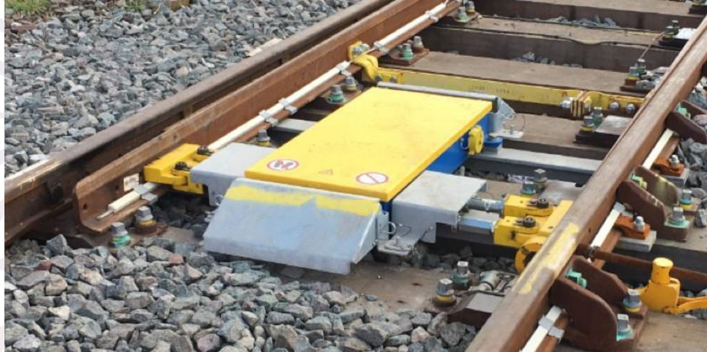
Figure 8 - Point machine installation
