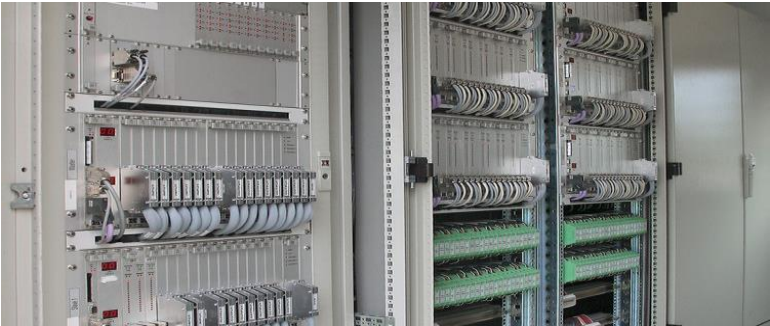
Figure 7 - Wall mounted internal location cabinet (undergoing factory testing)
